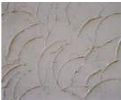
SKIP TROWEL STUCCO
