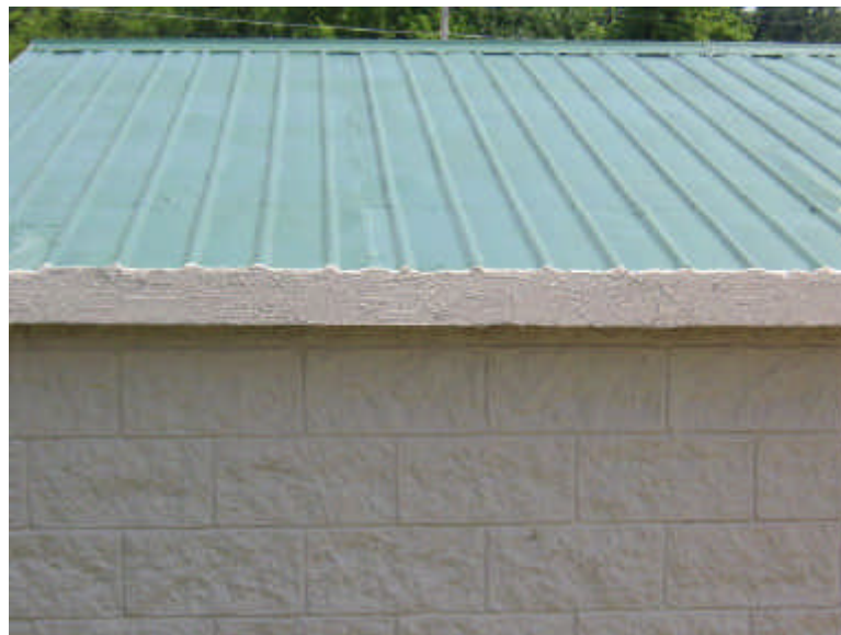
ROOF DETAIL SIMULATED RAISED SEAM METAL
